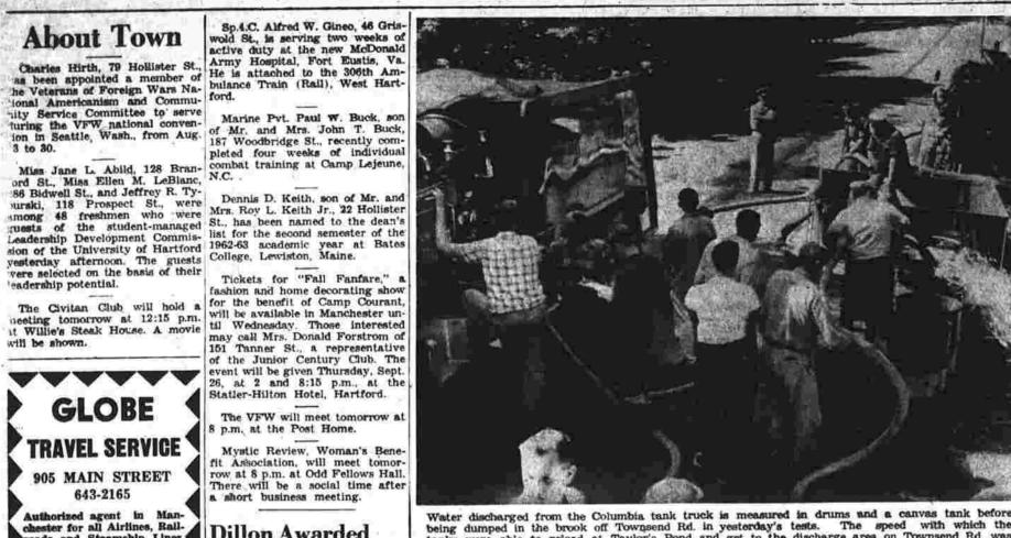
Water discharged from the Columbia tank truck is measured in drums and a canvas tank before being dumped in the brook off Townsend Rd. in yesterday's tests. The speed with which the tanks were able to reload at Taylor's Pond and get to the discharge area on Townsend Rd. was also carefully recorded. The Bolton pumper, in the right background, was used at the Townsend Rd. point; the Andover pumper at Taylor's Pond. (Herald photo by Paul D'Italia).
